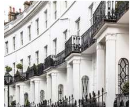
GROSVENOR CRESCENT HOUSE London, UNITED KINGDOM
