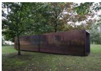
HOUSE + Lisbon, PORTUGAL
