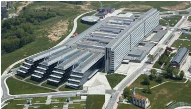
HOSPITAL UNIVERSITARIO CENTRAL DE ASTURIAS Asturias, SPAIN
